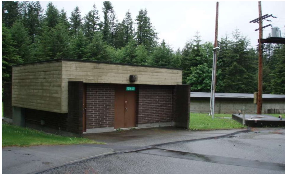
Figure 11: Water reservoir and pump station on 64 Avenue
