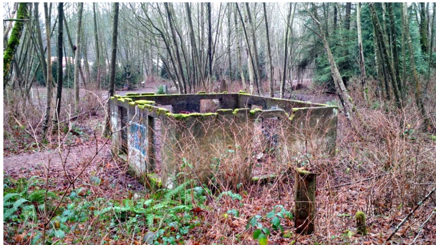
Figure 19: Original Well Pump House at Watershed Park, Constructed 1906
